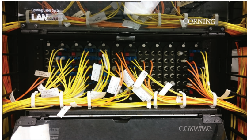
FIGURE 3-17 An example of a fiber patch panel.
